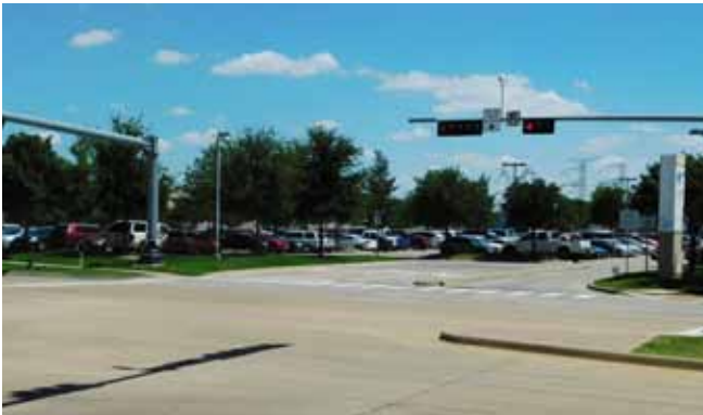
Located on light controlled street intersection with Dart Rail Station and large parking
